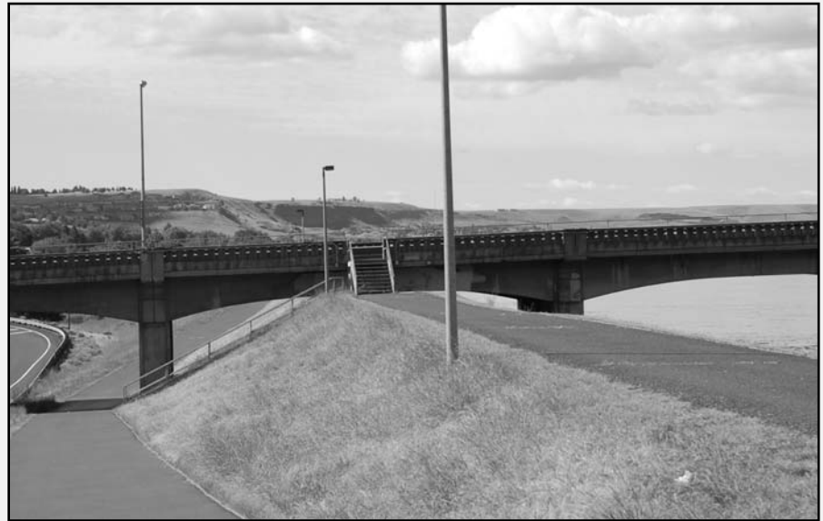
Sediment built up over the past 30 years since the Lower Granite dam was constructed have greatly reduced the ability of levees to protect the city of Lewiston in a high water year.
